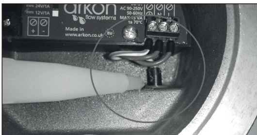
Pic. 2 Application of silicon binder on cable sheath of opened round cross cut cable end
